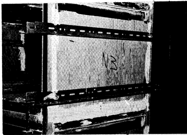
Figure 4 Formwork for Infill Wall
